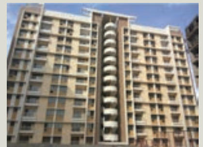
Construction of Phase-1 (Block-3)
