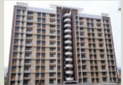
Construction of Phase-1 (Block-2)
