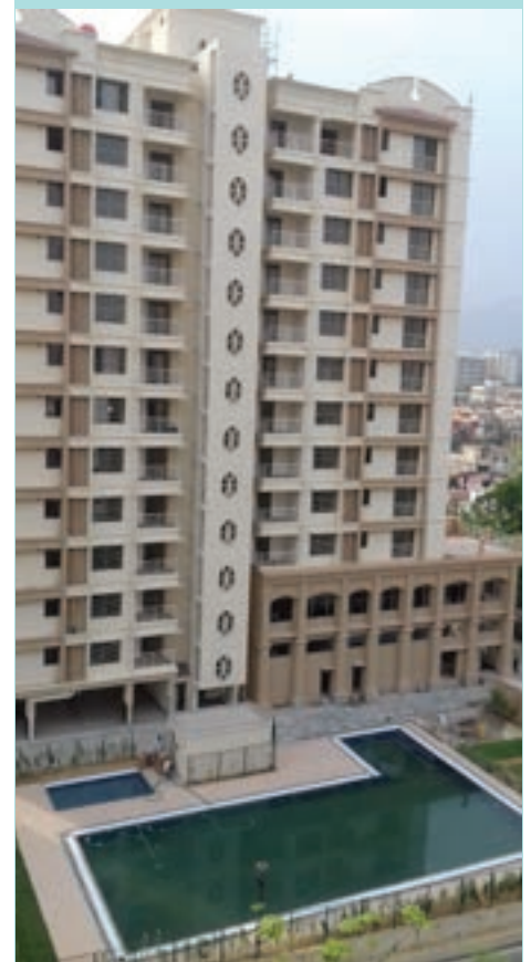
Work in progress of Aries Block, Club House and swimming pool
