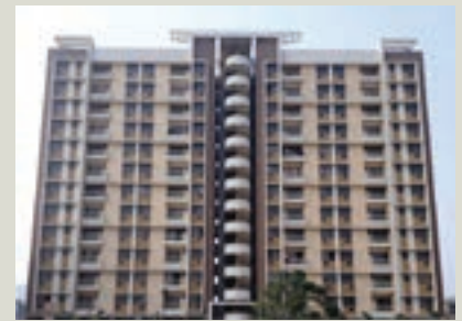
Construction of Phase-1 (Block-1)
