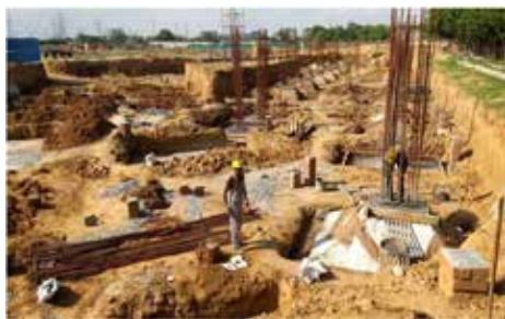
Foundation work of Bal Bharti Public School at Ashiana Town, Bhiwadi
