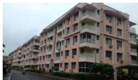
Exterior repairs and repainting at Ashiana Woodlands, Jamshedpur
