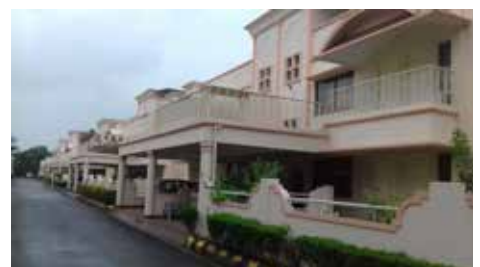
Ashiana Woodlands executive flats after repainting of exteriors
