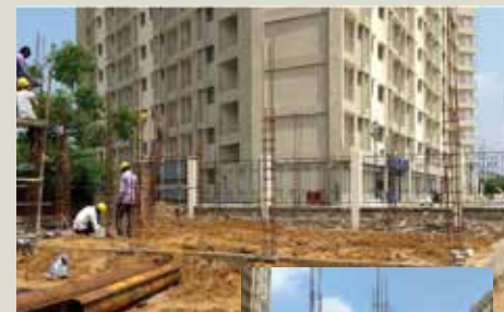
Construction work of Temple and Gate No. 2 at Ashiana Town-β, Bhiwadi
