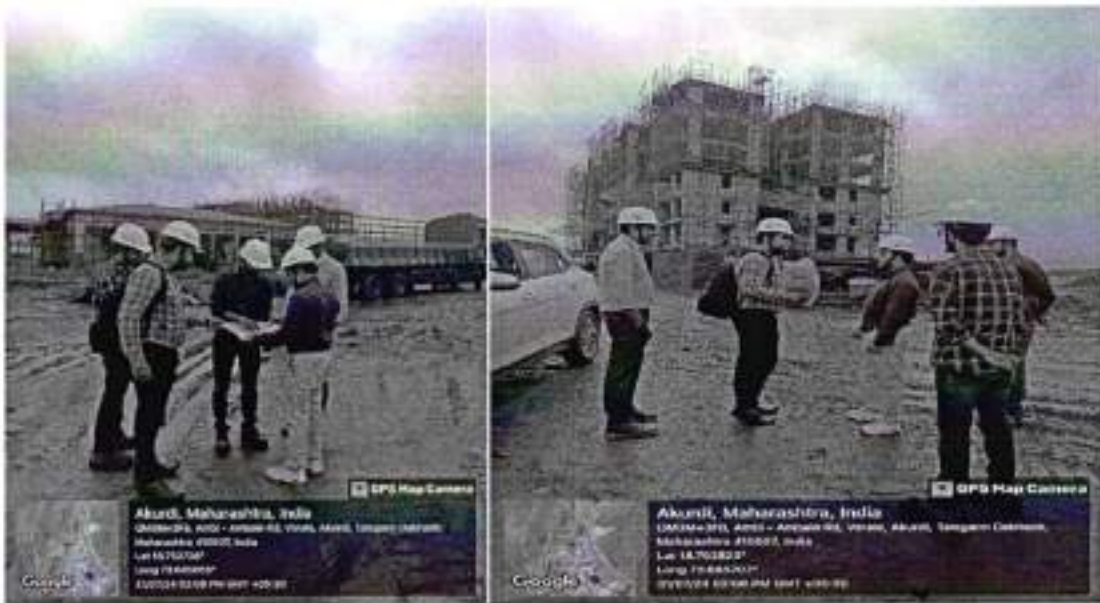
Fig. Construction at site
